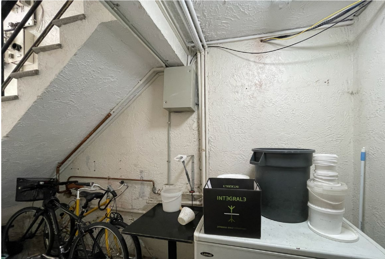
internal common residential stairwell
